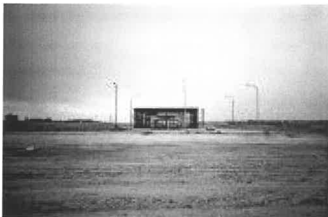
Figure 6: Madrid – Underground Station at MetroSur
